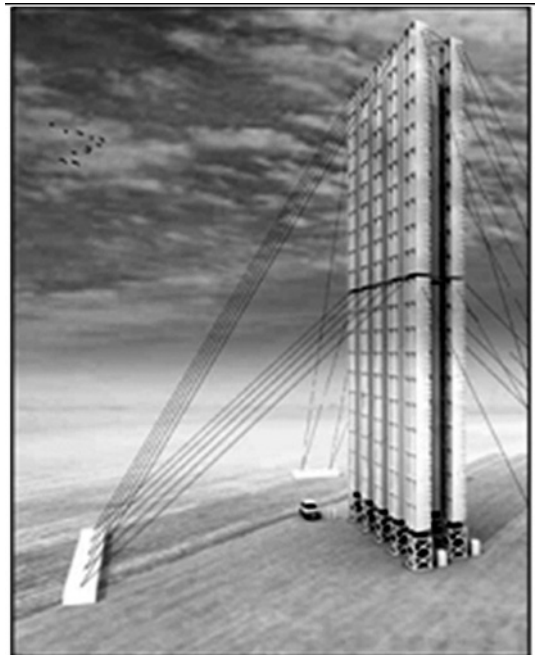
Fig. 2.3.2. Wind turbine farm is firmly anchored to the ground at multiple levels
