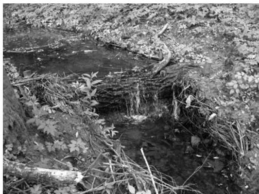
Fig. 6. Bottom weirs from wood in the Dorman creek valley
