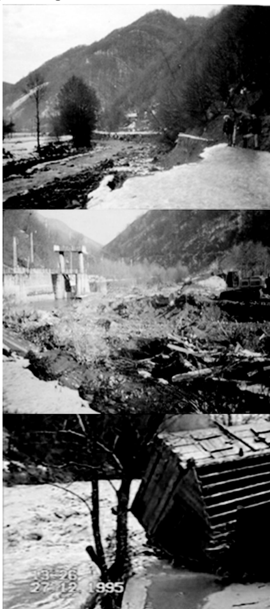
Fig. 6. Problems created by December 1995 floods in the valley of Someșul Rece; 1. Damaged road downstream of Maguri-Racatau; 2. Someșul Rece II intake plugged; 3. House driven by water
